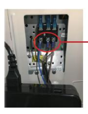
If the debugger is connected to the ODU terminal board, the communication wire of the IDU must also be disconnected.
